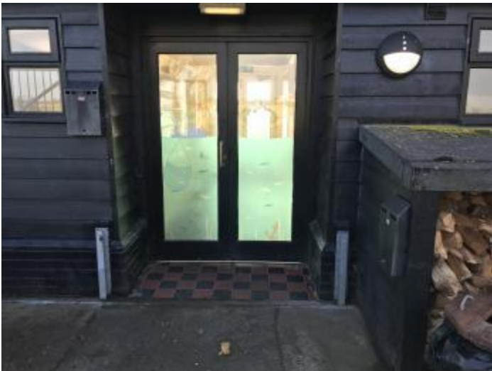
Rear Entrance Level Access
