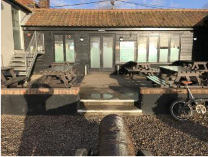
Main Entrance Exterior
