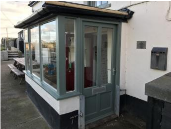
Rear Entrance With Step
